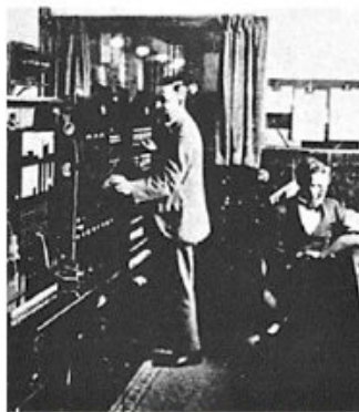
3LO Melbourne Control Room, 1925
