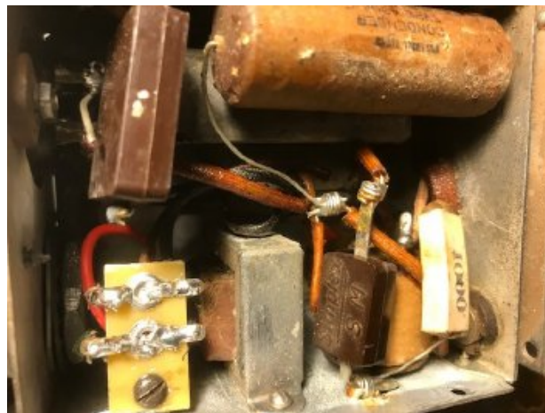
The 6v supply cables and all capacitors were replaced
