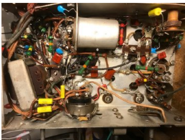
Airzone under chassis component wiring
